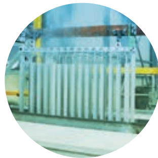
RAVAK plating plant Anodising aluminium profiles - manufacture of the sturdiest shower enclosure, door and bath screen frames.
